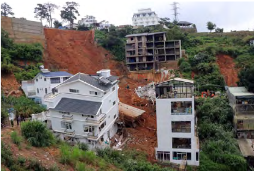
CI-DESSUS : PHOTO DES GLISSEMENTS DE TERRAINS RUE HOÀNG HOA THAM / ABOVE: PHOTO OF THE LANDSLIDES ON HOÀNG HOA THAM STREET
